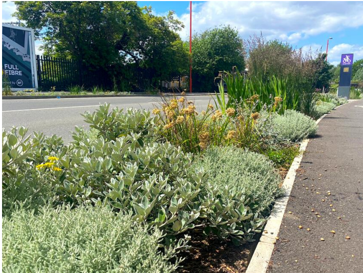
Forest Road, Meristem Design, Rain Gardens/ SUDs
